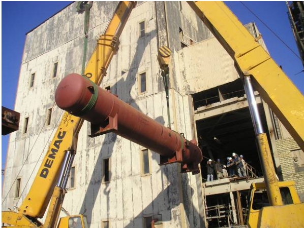
Hartha Heat Exchanger Replacement In Process
