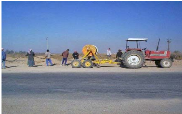
Cable Laying Along Baqubah - Khalis ITPC Backbone
