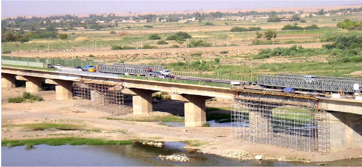
Tikrit Bridge Early in Construction
