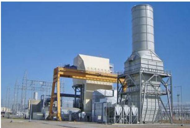
Completed Kirkuk v94 Power Plant
