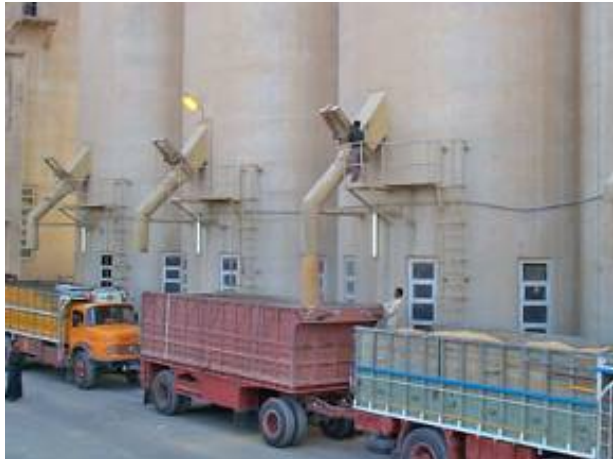
Grain Facility At Umm Qasr
