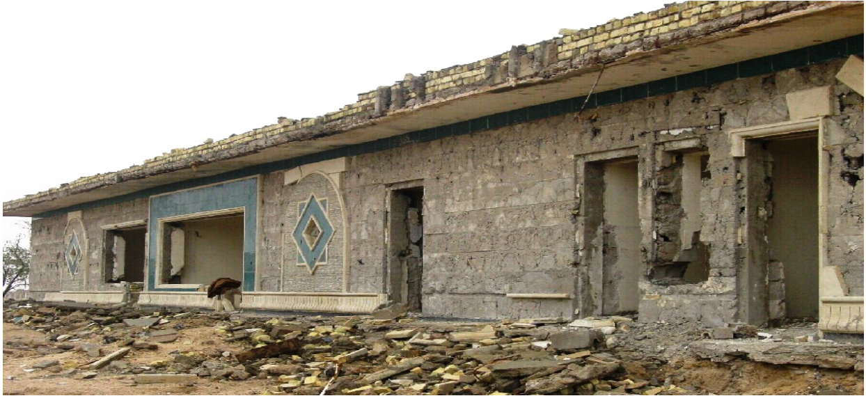
Typical Rail Station Before
