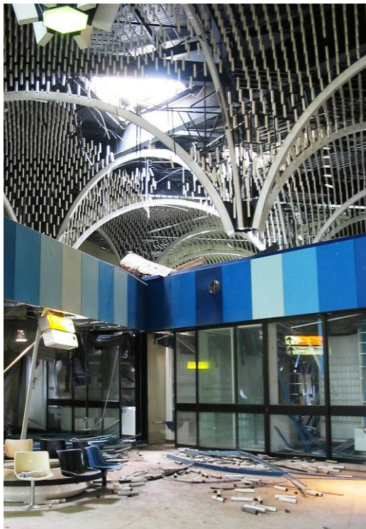
Baghdad International Airport roof damage
