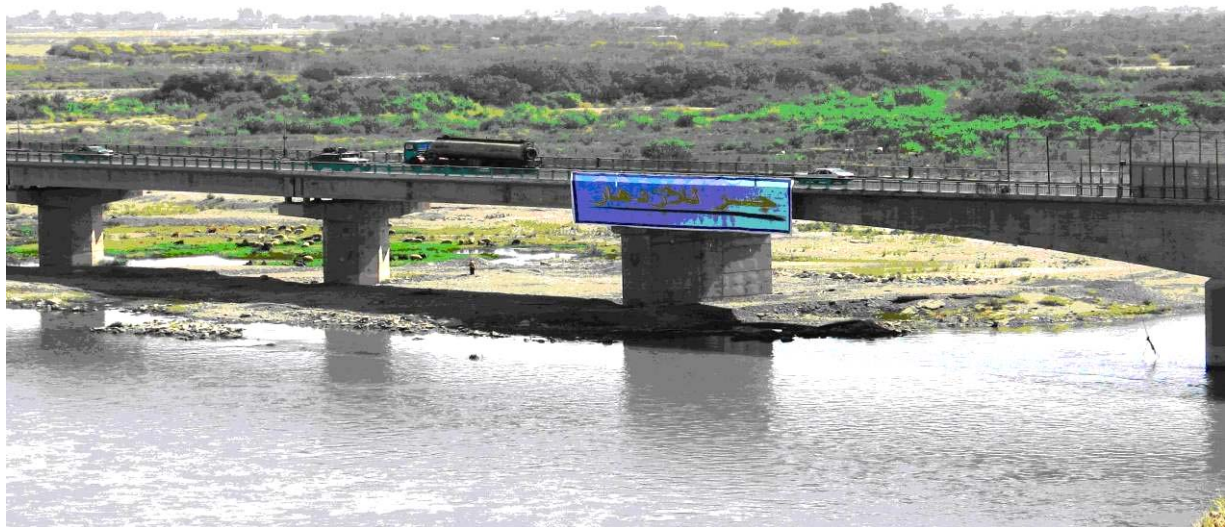
Tikrit Bridge Complete – Banner Reads “Bridge For Future Progress”
