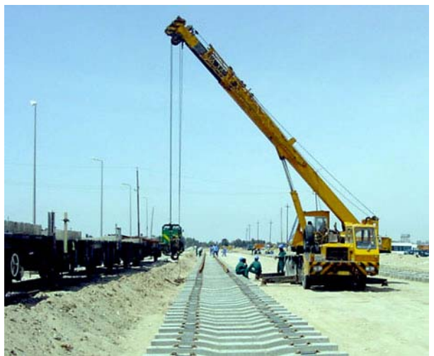
Laying New Track
