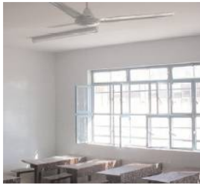
Typical Classroom After Restoration
