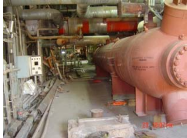
Hartha Heat Exchanger Installation Complete
