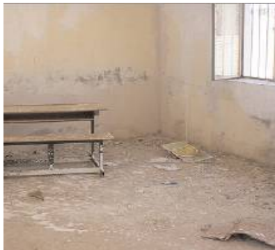
Typical Classroom Before Restoration
