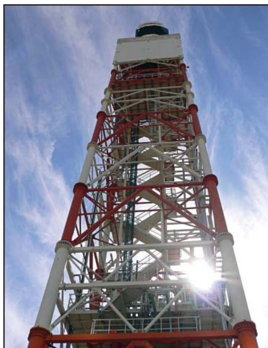
Figure 3. Solar Tower Installation
