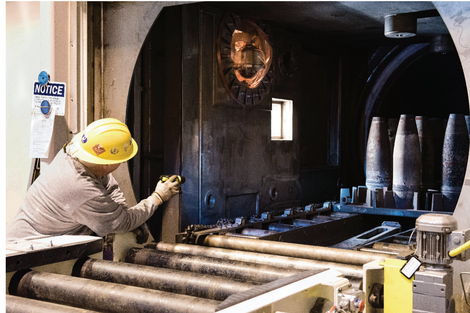
▲ Blue Grass Chemical Agent-Destruction Pilot Plant, Kentucky
