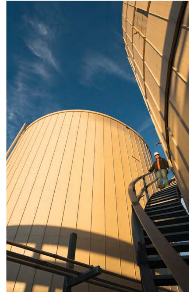
Chemical Agent-Destruction Pilot Plant Project-Pueblo, United States
