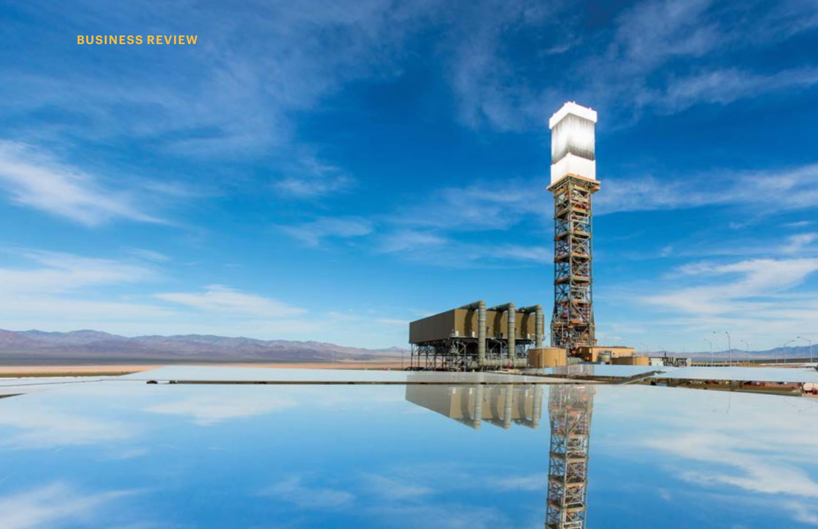
▲ Ivanpah Solar Electric Generating System California, USA
